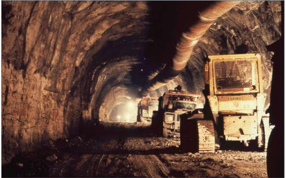
Darlington cooling water intake tunnel
