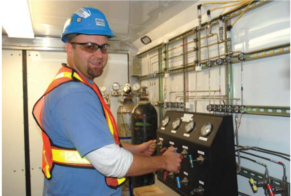
Borehole hydraulic testing trailer
